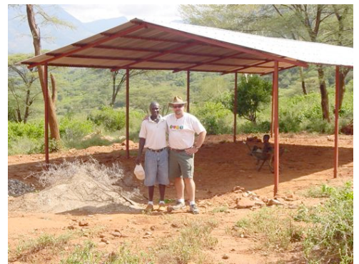
"Pilot" steel structure in Sigor
